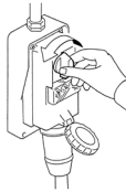
Position on “zero” the protection device placed upstream of the electric equipment feeding line.
